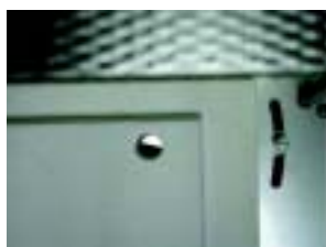
Inlet air opening in the door
