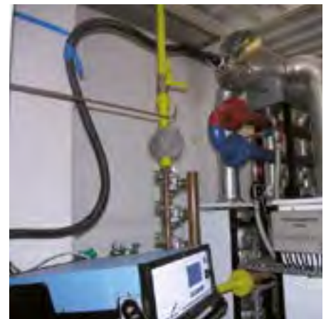
MONITORING OF COMBUSTION GASES ON INDUSTRIAL FURNACE
